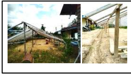
Figure 3. The side of the dryer building with a height of ± 100 cm
