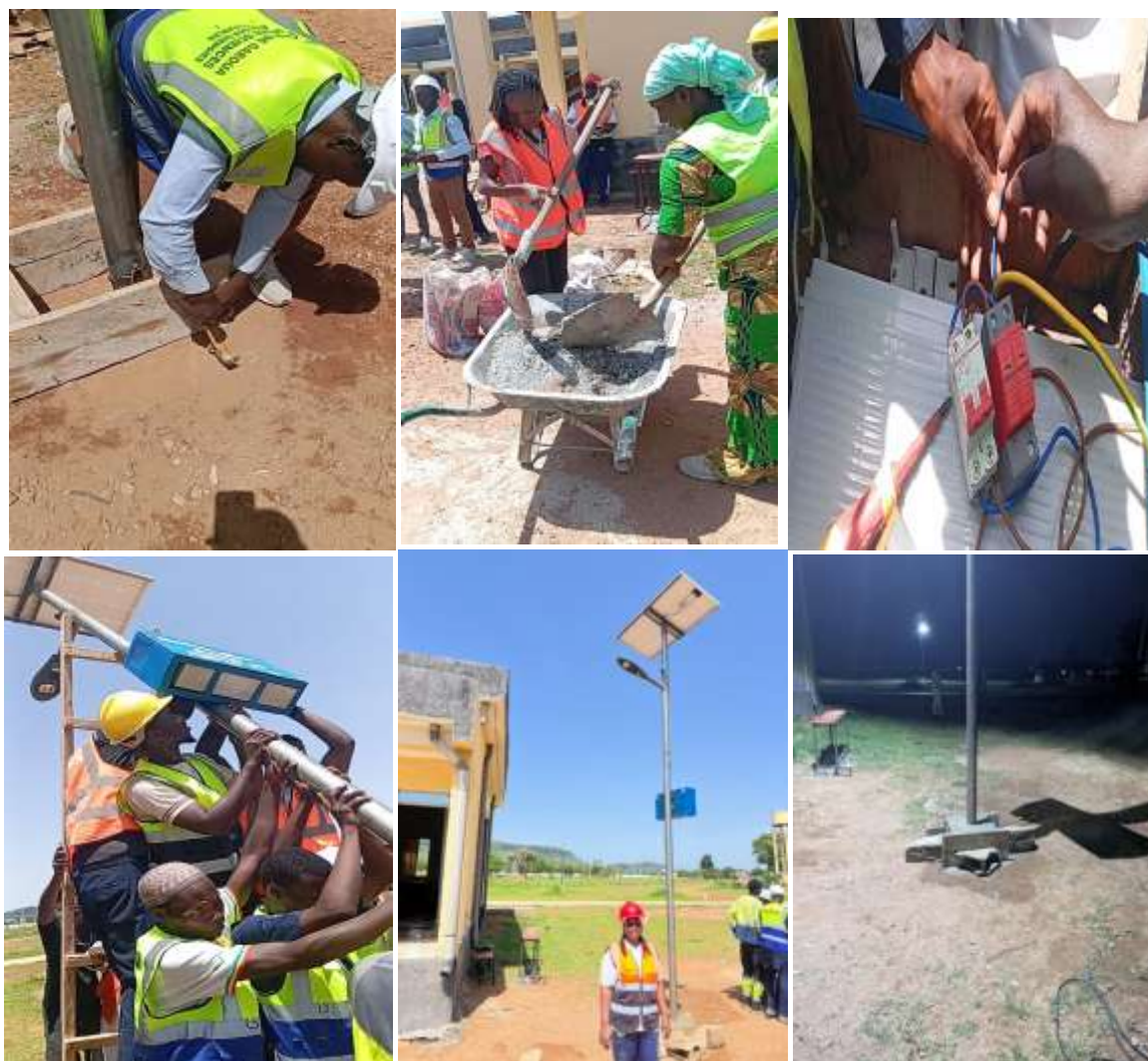
Figure 11: Some pictures of the installation stage.
