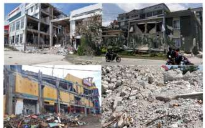
Figure 1. Damages of Structural Building after the 2018 Palu Earthquake and Its Debris (Sources: Author's Documentation)
