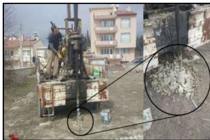
Figure 1. Drilling of a borehole for soil investigation.
