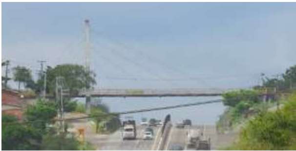
Fig. 1. Cable-stayed footbridge in Sergipe, Brazil
