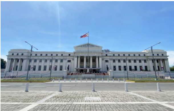
Figure 1.1 – Clean and treated facade of the National Museum of Fine Arts. Source: Google Images.
