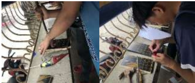
Figure II.-5. Drilling of holes in the base of the formworks
