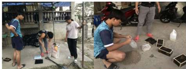
Figure II-9. Cement was prepared for concrete pouring
