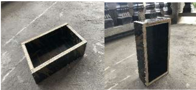
Figure II.-6. Assembling all the parts of the formworks
