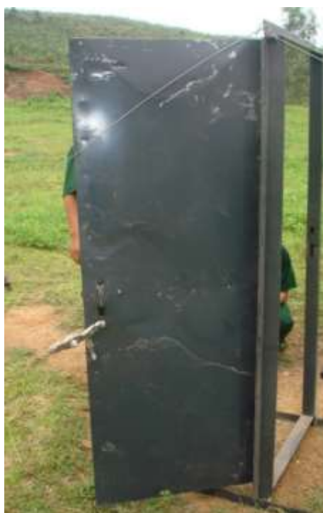
Fig. 13. Door-lock system after explosive loading
