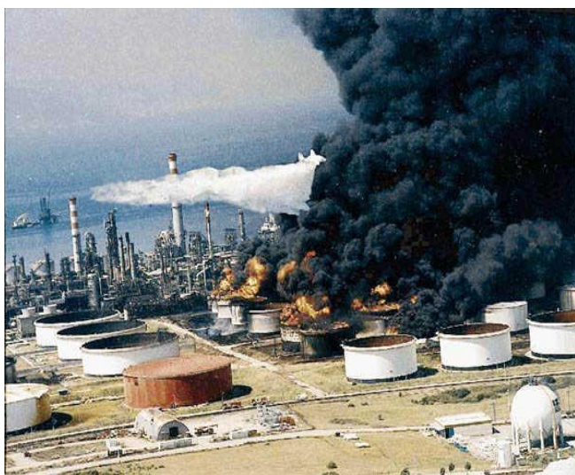
Figure 1. Aerial view of Tupras refinery after the Kocaeli earthquake (Turkish press, 1999)
