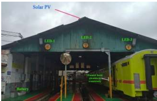
Figure 7. Spatial distribution and component configuration of the integrated solar-powered signaling system at the maintenance depot
