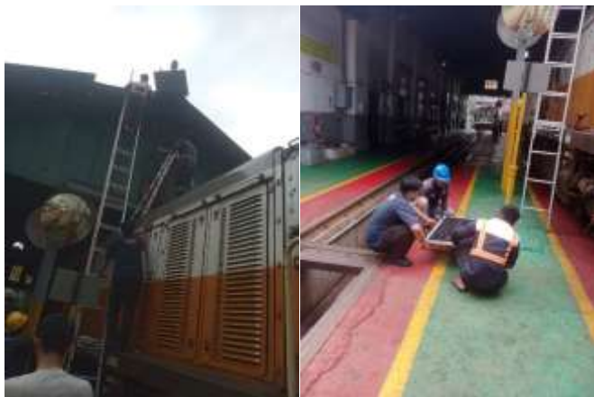
Figure 6. Installation of photovoltaic panels on the roof of the railway maintenance depot
