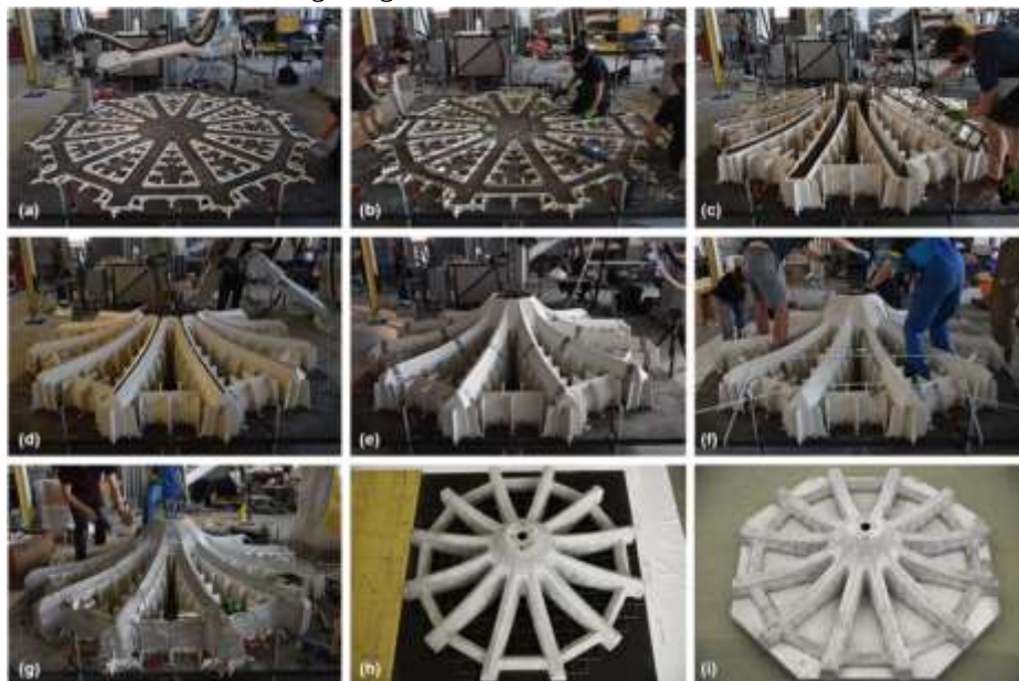
Figure 3: Fabrication steps of the prototype. (a) 3D Printing bottom 35 mm, (b) placing slab reinforcement, (c) placing rib reinforcement cages, (d) 3D printing cap formwork, (e) 3D printing column-slab transition, (f) casting of rib formwork, (g) demoulding of ribs, (h) cast and demoulded ribs, (i) complete slab prototype after casting of the solid part of the slab (Burger, et al., 2022).
