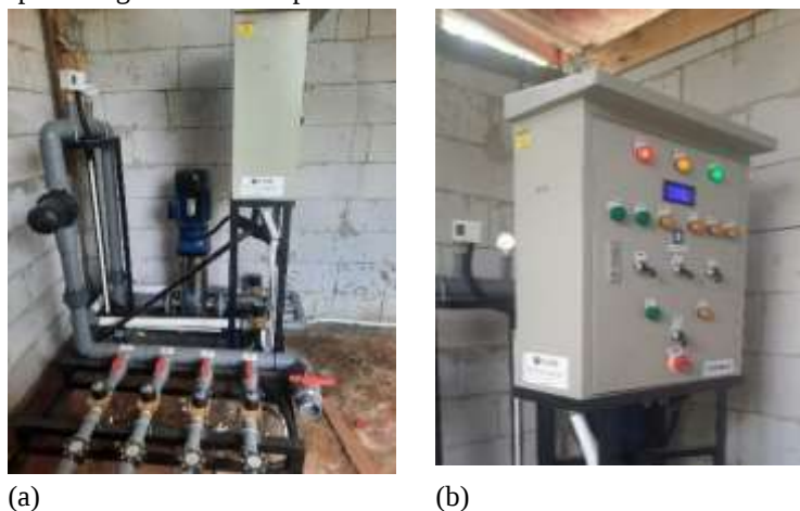
Figure 5 Cassmatech module (a) pump installation module and integration, (b) device testing (automatic and manual mode)
