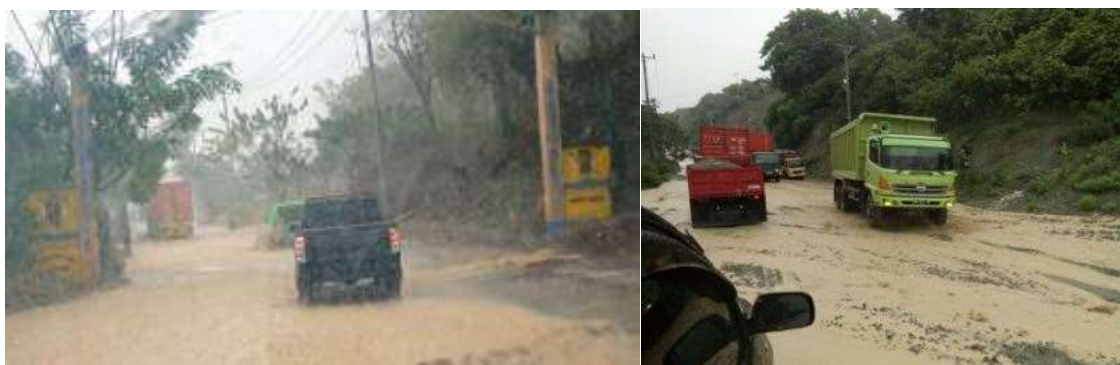
Fig.7 Condition of the Palu-Donggala road during the rainy season
