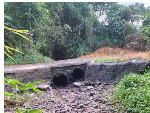
Figure IV-IV Existing Pipe Culvert Bridge
