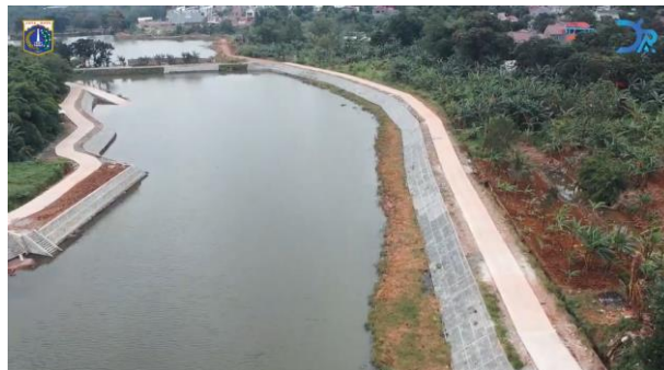
Figure 1. Construction of the Cilangkap Reservoir 2022
