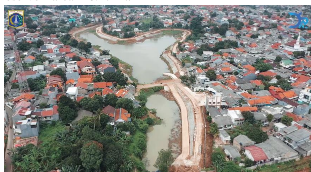
Figure 3. Construction of the Munjul Reservoir 2022
