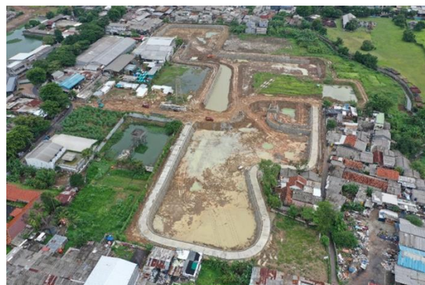
Figure 2. Construction of the Aseni Reservoir 2022
