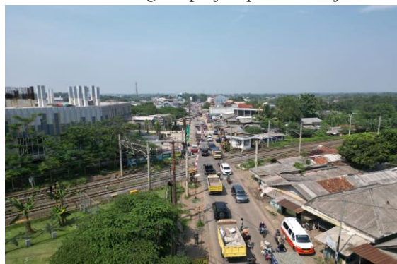
Figure 1. Initial Condition of Work
