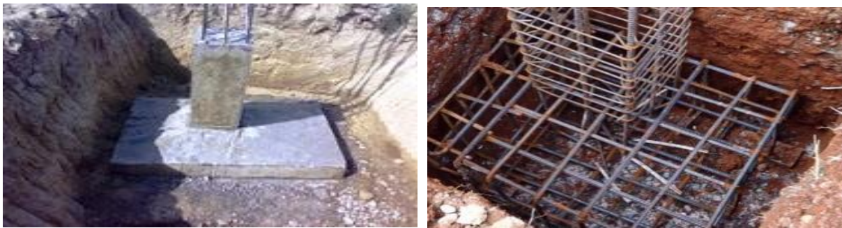
Fig. 1. Implementation of casting without a work floor
