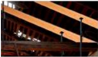
Figure 4. Remaining parts of the rafter V-shape wedge extension ((Abramyan & Ishmametov, 2016)
