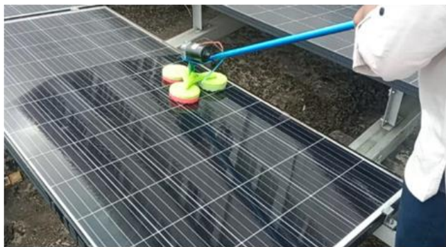
Figure 15. Process for cleaning solar panels using the wet method
