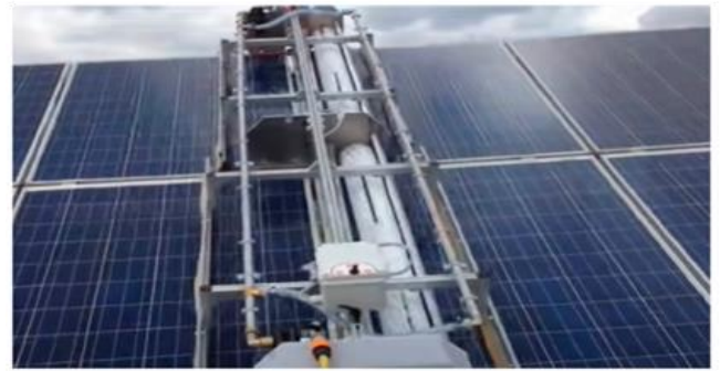
Figure 1. Solar panel cleaning robot with brushing system (Najmi et al., 2023).
