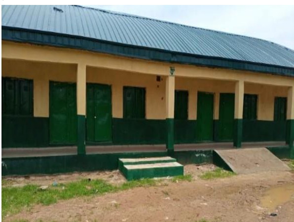
Fig.2: a. Ramp on class Building at Nagari
