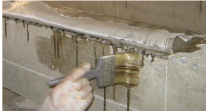
Fig 2. Application of epoxy resin
