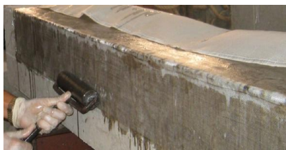
Fig 4 Removing air bubbles with the help roller
