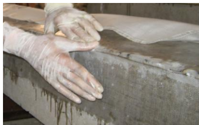
Fig 3 Fixing of GFRP sheet
