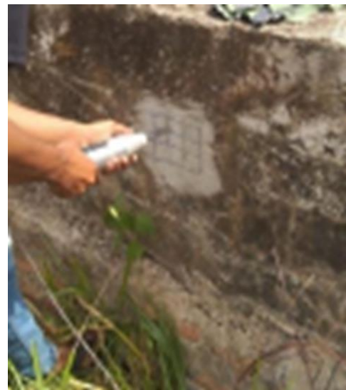
Figure 14. Process of testing sloof concrete hardness using a hammer test
