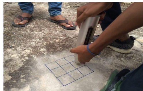
Figure 15. Process of testing floor plate concrete hardness using hammer test
