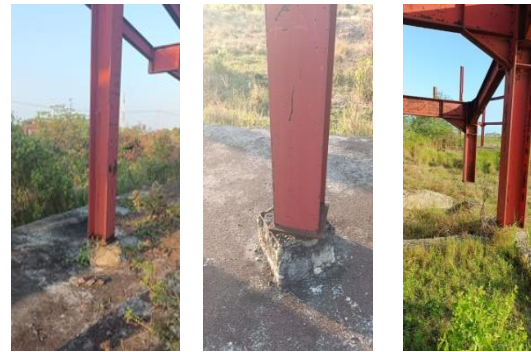
Figure 2. Column placement on the pedestal
