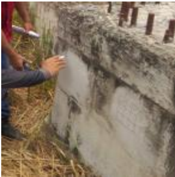
Figure 13. Pedestal column concrete hardness testing process
