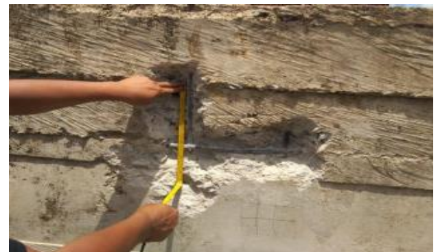
Figure 9. Measurement of reinforcement distance
