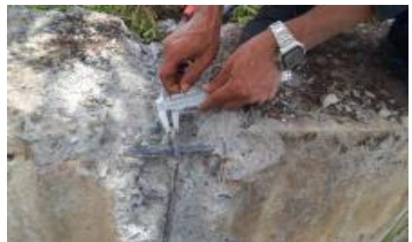
Figure 11. Measuring reinforcement diameter with a sigmat tool
