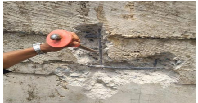
Figure 8. Concrete breaking process
