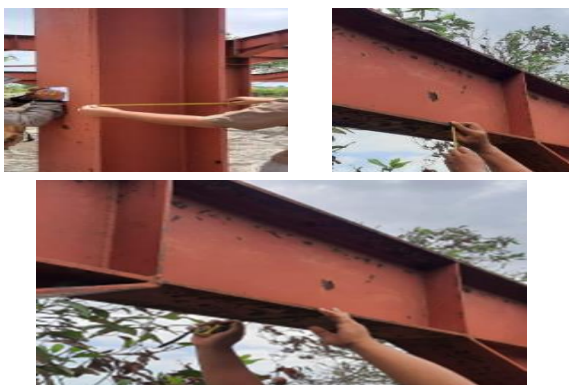
Figure 7. Measurement of steel columns and beams
