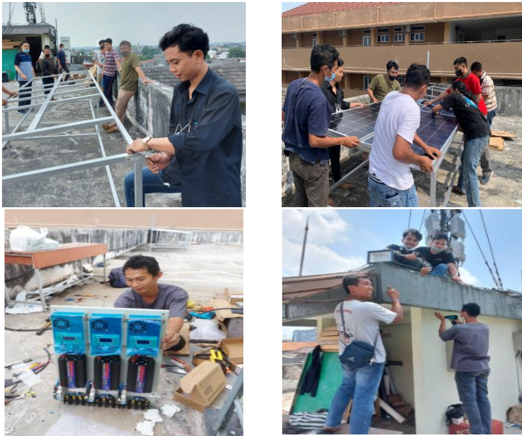
Fig. 1. Photograph of installation work
