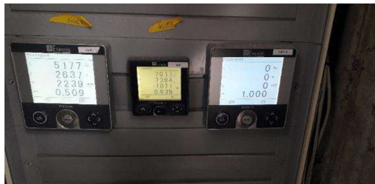
Figure 4. Measurement units (in the middle) and Control units + concentrator with display (on the right and on the left)
