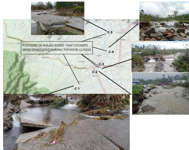
Fig. 4.1. Location and evidences of culverts that were devastated by Typhoon Ulysses
