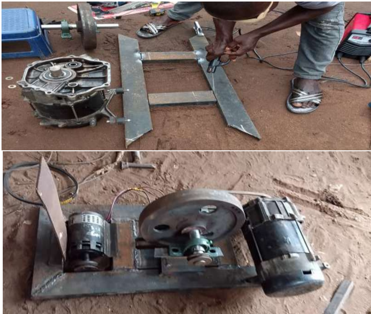
Figure 7: Fabrication of the 5 KVA Fuel
